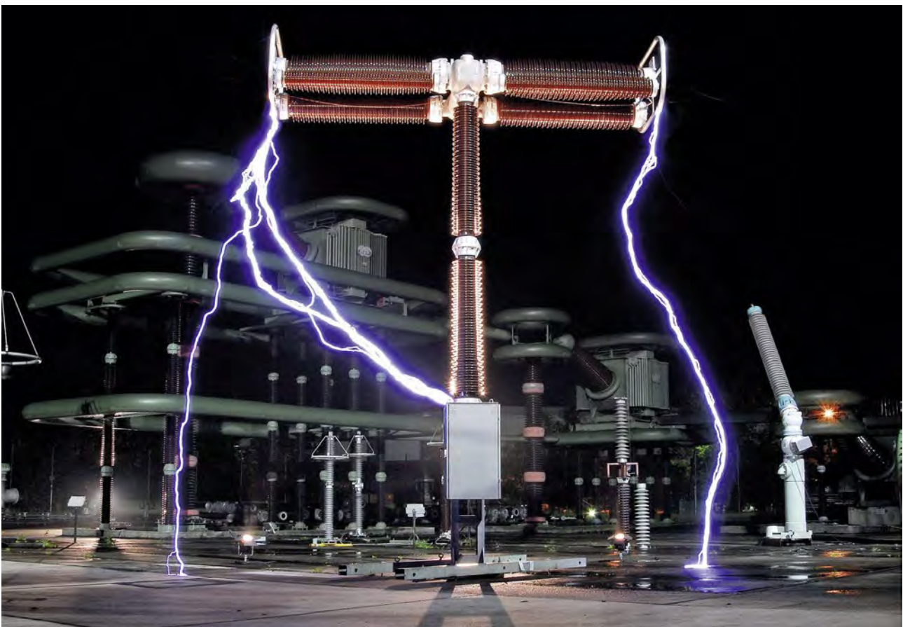
Fig. 1/3: Internal arc during an overvoltage test in the Siemens Switchgear Plant Berlin
